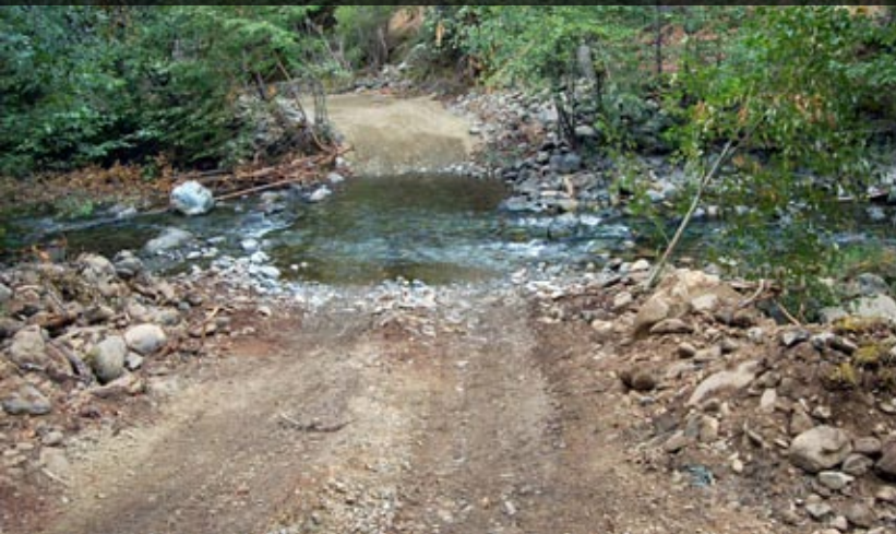
GEORGE SEXTON (KSWILD) Roads carved through creek beds and turbid water collected in holding ponds were just part of the illegal mining operations at Sucker Creek in 2009.
